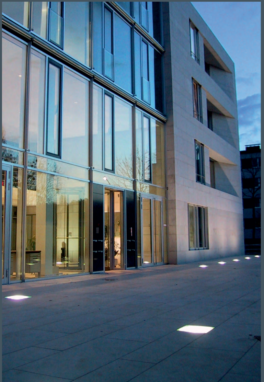
Ground-recessed luminaires with asymmetrical or wall washer reflectors produce uniform façade illumination.
